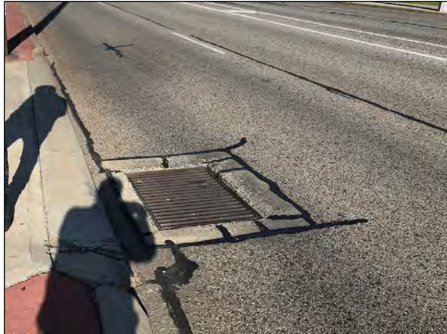
Finding 2.5 – Lack of on road cycling facilities, narrow traffic lanes and non-compliant stormwater grates.
